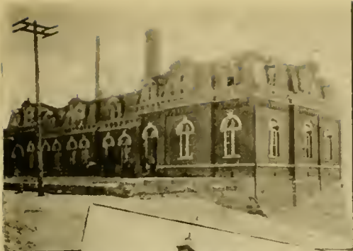
CITY WATER WORKS
